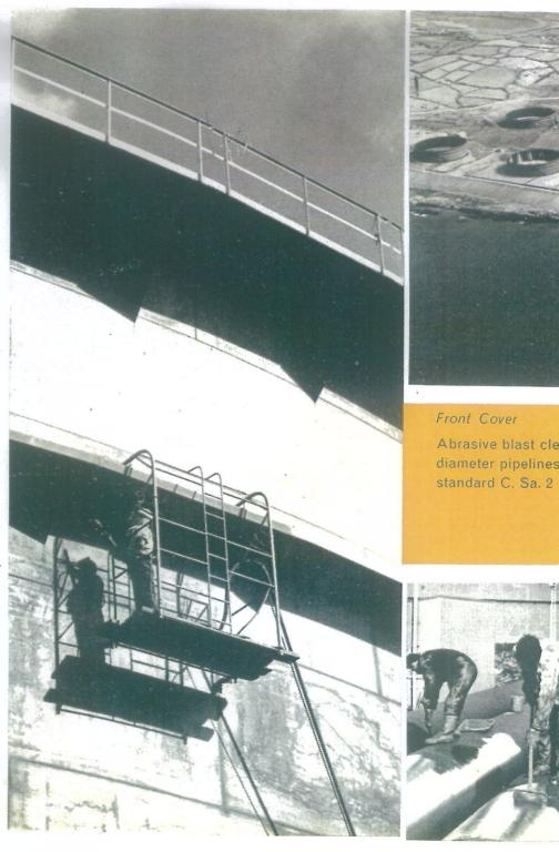
Abrasive blast cleaning c diameter pipelines to Swe
